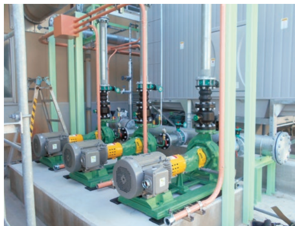
Manufacturing facilities at the Fukushima No. 1 Factory
