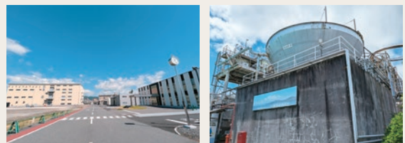
A panoramic view of the factory and the wastewater treatment facility.
