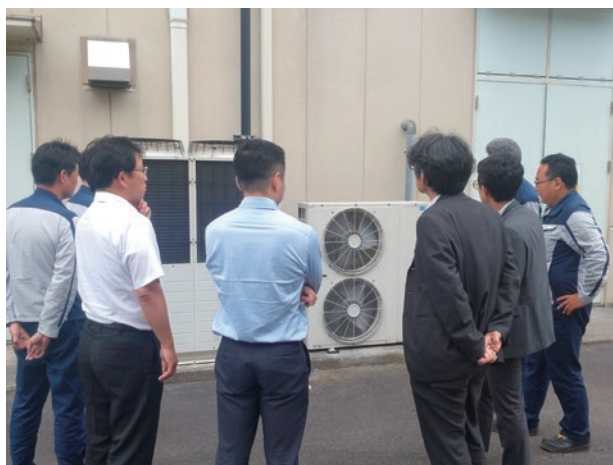
Viewing an outdoor air-conditioner unit in front of an office
