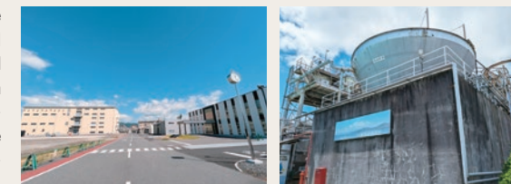
A panoramic view of the factory and the wastewater treatment facility.
