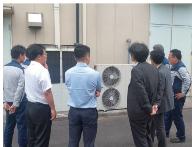
Viewing an outdoor air-conditioner unit in front of an office
