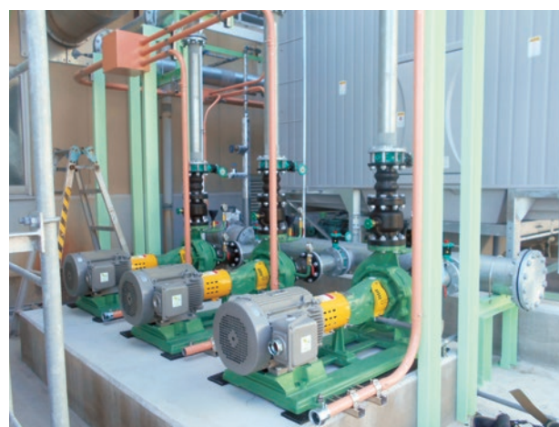
Manufacturing facilities at the Fukushima No. 1 Factory
